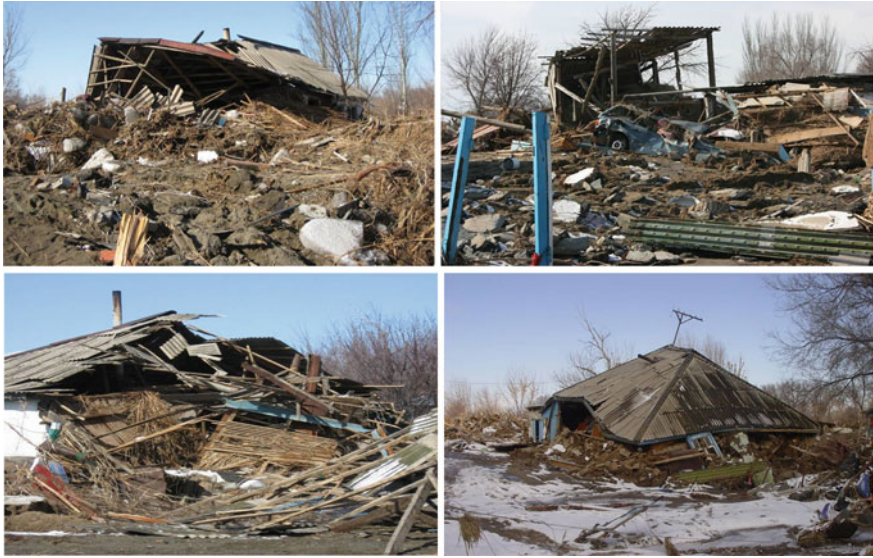
Fig. 2 Consequences of flooding disaster in the village of Kyzylagash
